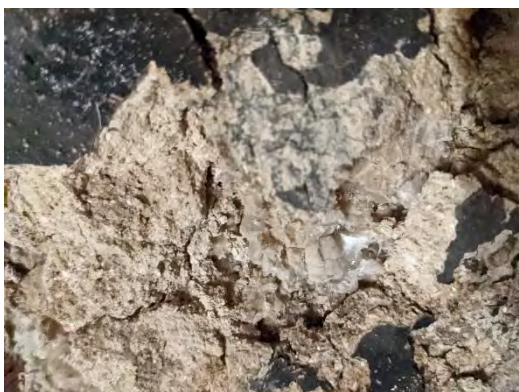
>> Figure_4.2.03. Crystallization of salt deposits in rock, fragment of the ceiling of the northern chamber [Q] Photo // Dmitry Petrenko
